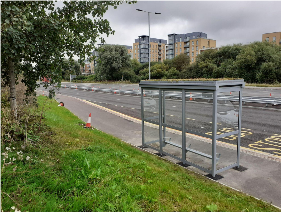
A ‘green roof’ bus shelter being trialled to improve urban air quality and biodiversity on the A33 corridor in south Reading.
